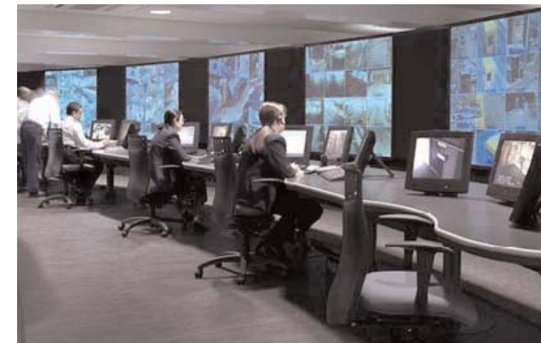
NCP Control Room, Manchester
